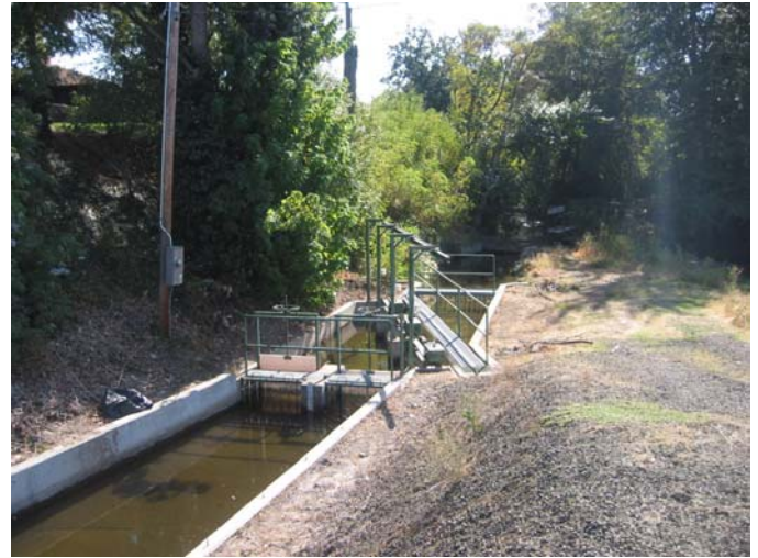
Eastside Diversion – Fish screens
