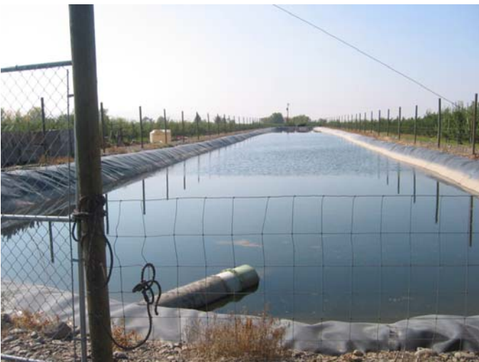
Brown & Sons – Bulge
